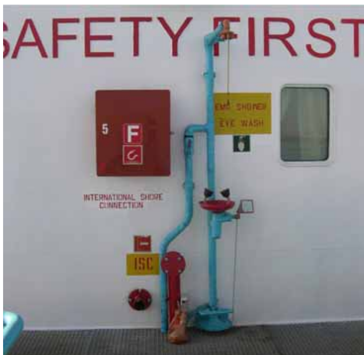
Photograph 3.3 - Decontamination Shower and Eyewash Station
